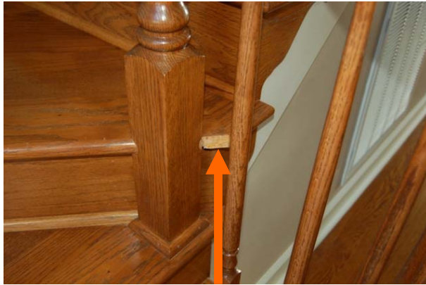
Chip on edge of step
