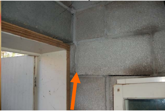
Typical crack
