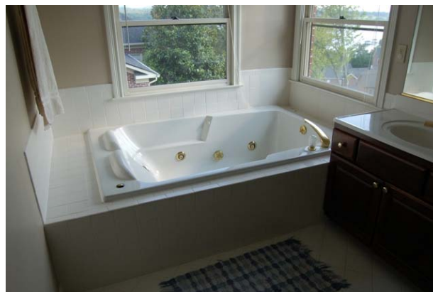
No access panel
